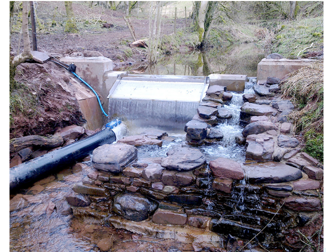
Above: the intake for one of TGV Hydro's micro hydro schemes, shortly after completion. Photo: TGV Hydro Ltd.
